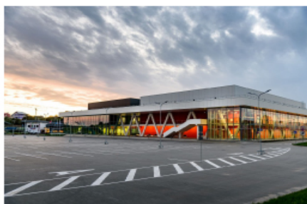
Sports Complex Rezekne Sports Complex Rezekne, Latvia Developer: Rezekne City Council Architect: REM PRO Ltd
